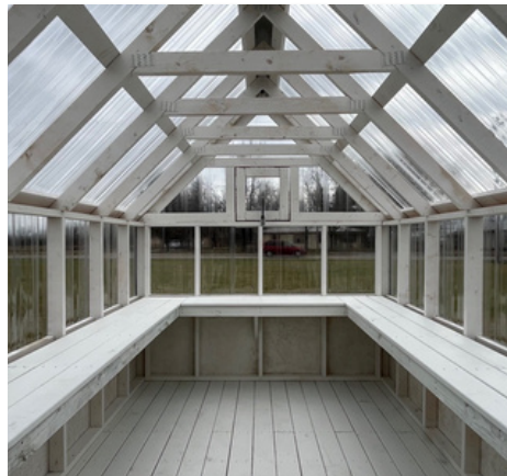
Deck-board potting shelf around the perimeter (sides and back wall)
