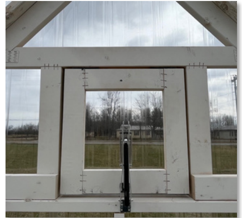
Vent door with Automatic Opener (opens between 59-77°F)
